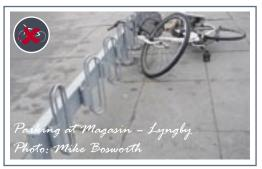
Bad rack which does not "grip" the front wheel sufficiently well. The stand is model 51 GE from Veksø.
