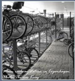
Notice the solution which means that the lower parking deck is set below the access level. This reduces the lifting which it takes to park a bicycle in the upper deck.
