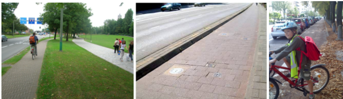
Cycle paths with verge partition, kerb partition and behind a parking lane (image source: T. Aspergers, P. Kroeze, D. Dufour)
