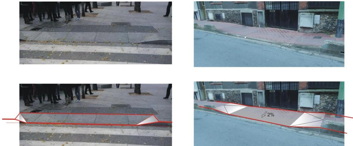
Figure 5 – **Perpendicular curb ramp** (left) **Parallel curb ramp** (right) (Source and editing: O. Stepan)
