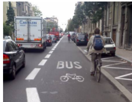
A tight bus/bike lane helps to bypass a congestion point, with an open profile and cycle symbols (D. Dufour)
