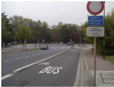
Bus/bike lane as a traffic light bypass for a right turn, with a closed profile and cycle road symbols (D. Dufour)
