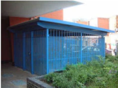
Secure and visible external cycle storage for flats Portsmouth, UK image source: Cycling England, Tony Russell
